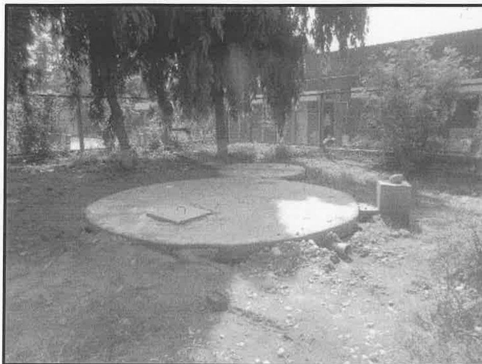
Rain water harvesting structure
