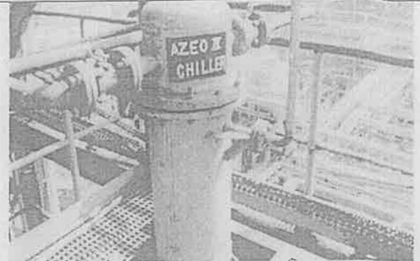
Chiller to reduce the emission so as to reduce vent losses from the tank
