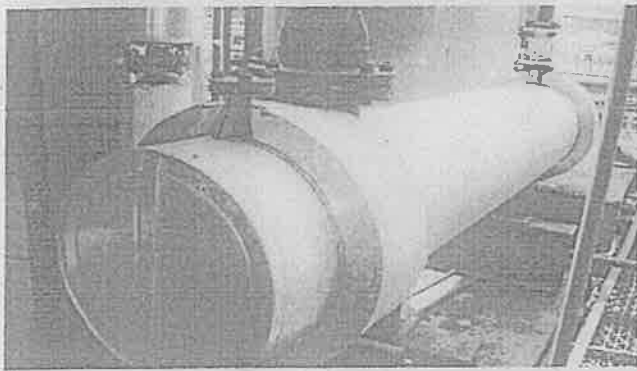
Chiller to reduce the emission so as to reduce vent losses from the tank
